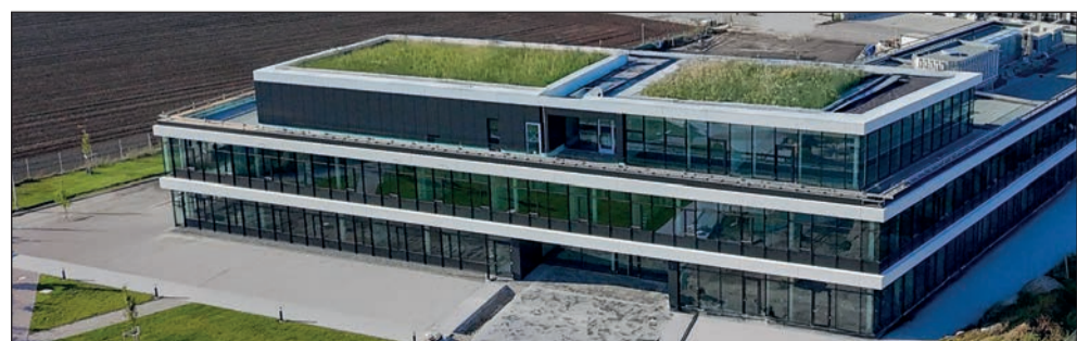
Most recent in this growth strategy has been the expansion of the company’s headquarters in Munich, considered to “symbolise” GROUP7’s long-term commitment
